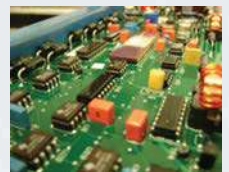
Battery Management System (BMS)
