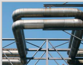
Pipelines subject to pressure
